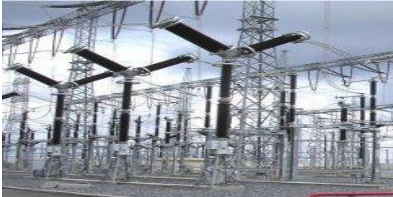
Gambar 2.7 SF 6 Circuit Breaker
