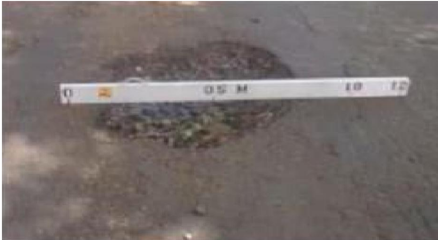
Gambar 2.29 Lubang (Pathole)
