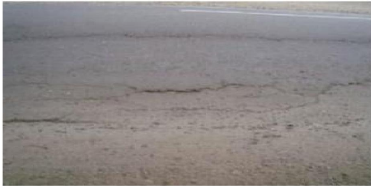
Gambar 2.11 Cekungan ( Bump and Sags )
