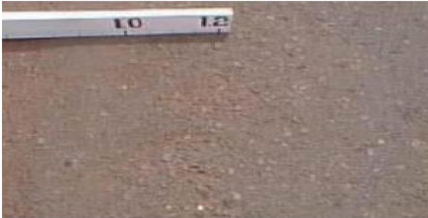
Gambar 2.27 Pengausan Agregat ( Polised Agregat )
