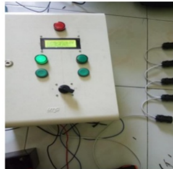
Gambar 19. Kontrol Switch keadaan Solar Cell ON
