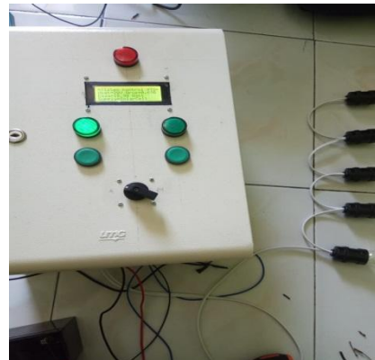
Gambar 19. Kontrol Switch keadaan Solar Cell ON
