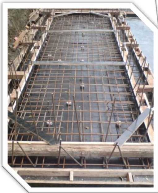
3. Moulding Slab
