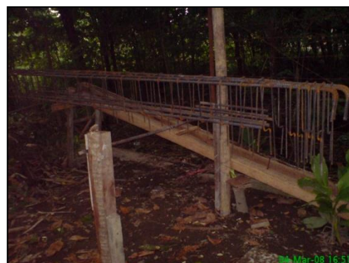
Area Kerja Besi
