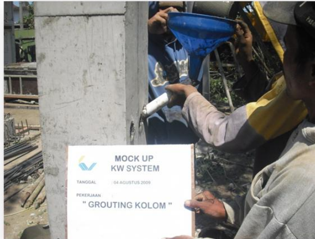
Grouting Kolom
