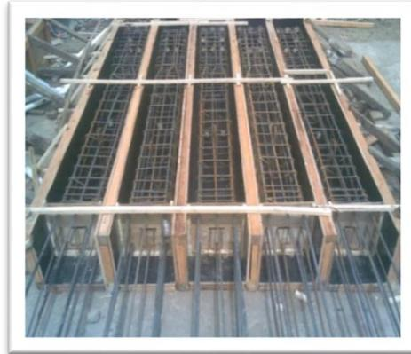
**Gambar 2.3.** *Moulding/cetakan Kolom*
