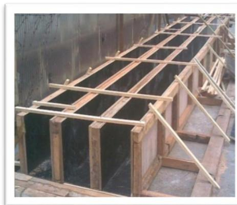
**Gambar 2.4.** *Moulding/cetakan Balok*
