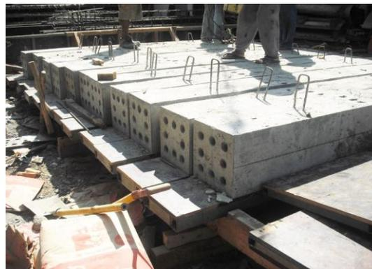
**Gambar 2.10.** *Stacking Beton Precast*
