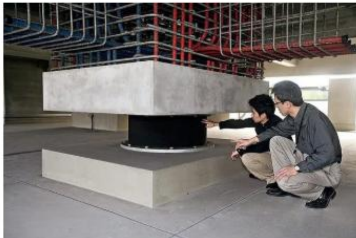
Illustration of HDRB when installed
