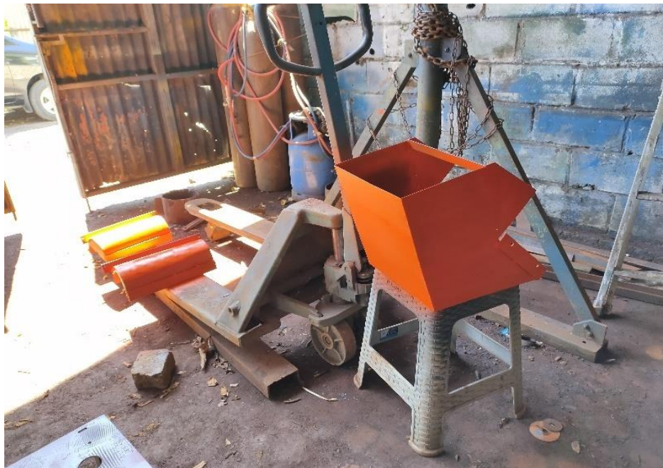
Proses pengecatan casing belt conveyor.
