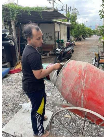
Putting all the sand and gravel into the molen
