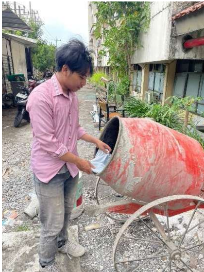
Putting cement and bamboo leaf ash into the concrete mixer.
