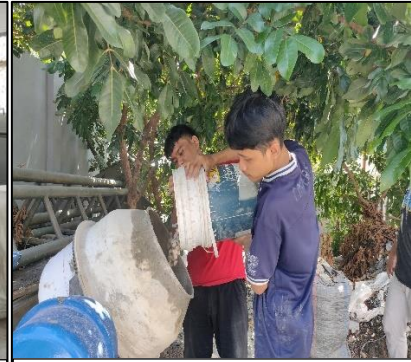
Putting material into the mixer
