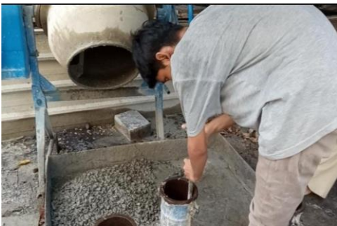
Stabbing concrete in the mold
