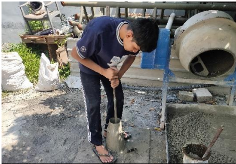
The process of slump test
