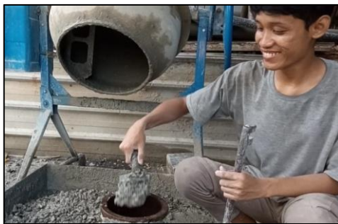
Putting concrete into the mold
