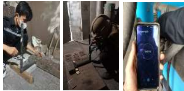
Gambar 3. 2 Persiapan Proses manual sandblasting
