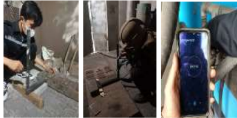
Gambar 3. 2 Persiapan Proses manual sandblasting
