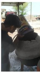
6. After the material is put into the mixer, turn on the mixer so that the mixer can move. After a few minutes add water and pour it into the mixture in the mixer, then after some time, put the superplasticizer into the mixture and add more water until the concrete mixture looks all mixed. The time required for the concrete mixture to mix all ± 20 minutes.
