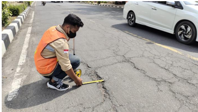
Calculation of The Width of The Damage (Source : Reseacher Data, 2022)
