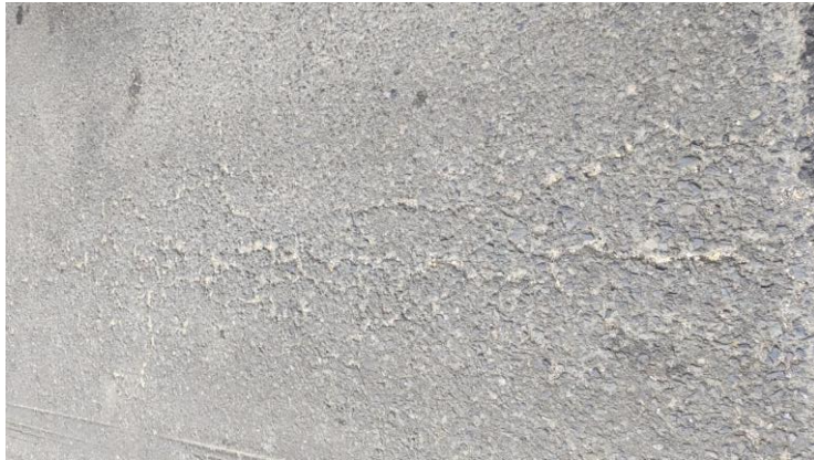
Figure A 5 Ravelling (Source : Reseacher Data, 2022)
