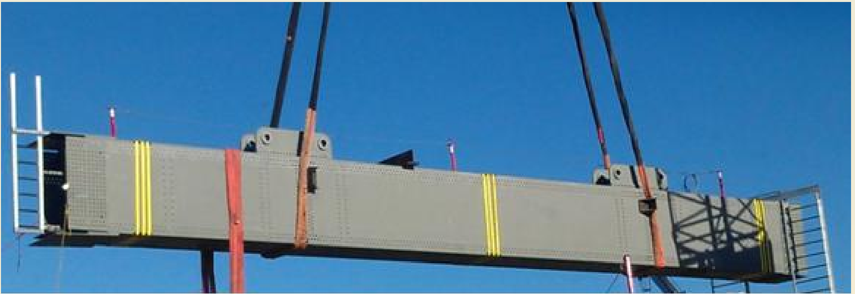
Erection of Girder
