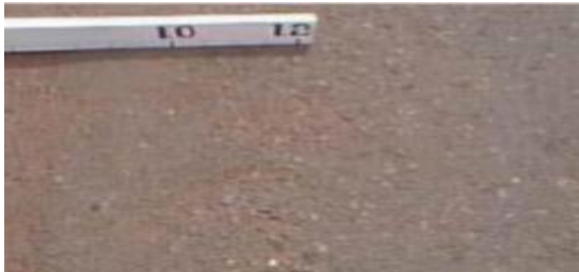
Gambar 2.14: Pengausan Agregat (Polished Agregat)
