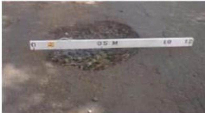
Gambar 2.12: Lubang (Pothole)
