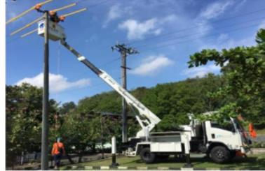
Gambar 4. 2 PDKB Sentuh Langsung (Contact Method)
