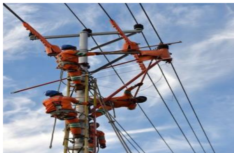
Gambar 4. 1 PDKB Berjarak ( Distance Method )
