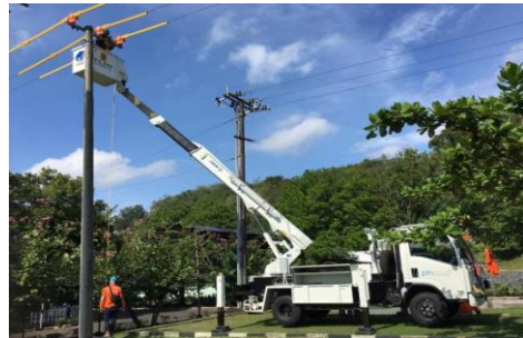
Gambar 4. 2 PDKB Sentuh Langsung ( Contact Method )
