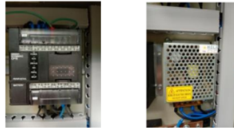
Gambar 4.2.4 PLC Omron dan Power Supply
