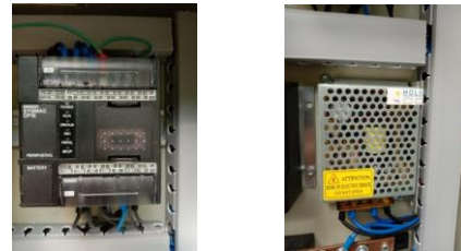
Gambar 4.2.4 PLC Omron dan Power Supply
